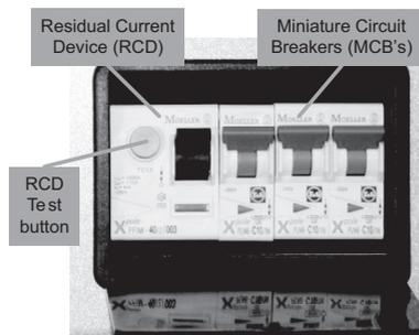
The Residual Current Device (RCD) is basically provided to protect the user from lethal electric shock. The RCD will turn off (trip) if the current flowing in the live conductor does not fully return down the neutral conductor, i.e. some current is passing through a person down to earth or through a faulty appliance.
