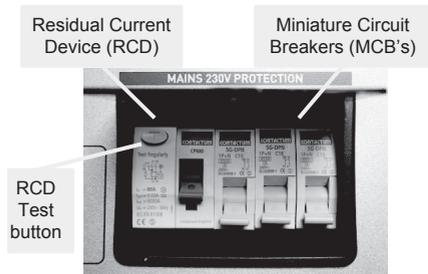
The Residual Current Device (RCD) is basically provided to protect the user from lethal electric shock. The RCD will turn off (trip) if the current flowing in the live conductor does not fully return down the neutral conductor, i.e. some current is passing through a person down to earth or through a faulty appliance.
