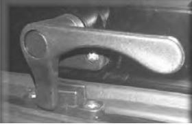
The retaining catches are as previously described on side window catches and can also be positioned to night vent.
