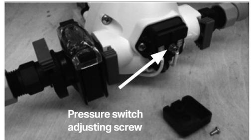
The pump may have to be removed to gain access to the adjusting screw. Drain the water system before removing the pump. To remove the pump pull the blue taps at right angles to the pipe work and lift the pump out.
